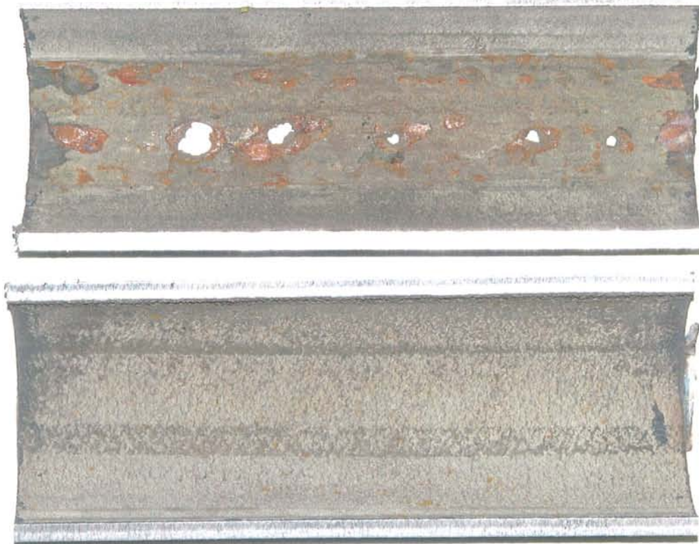
Figure 12 Internal Surface of Section #6
