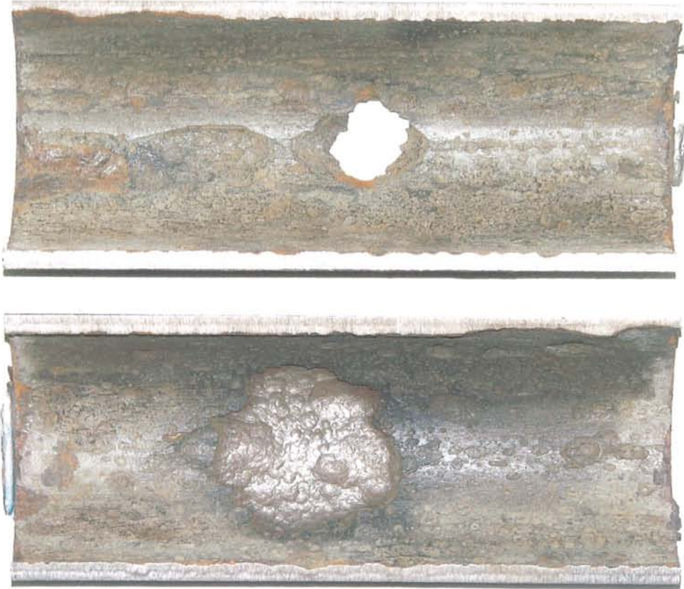
Figure 5 Internal Surface of Section #2 After Cleaning
