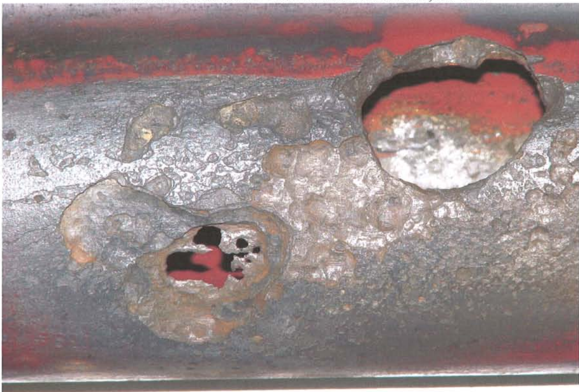
Figure 19 External Corrosion on the Gas Lift Mandrel from 3,860 Feet
